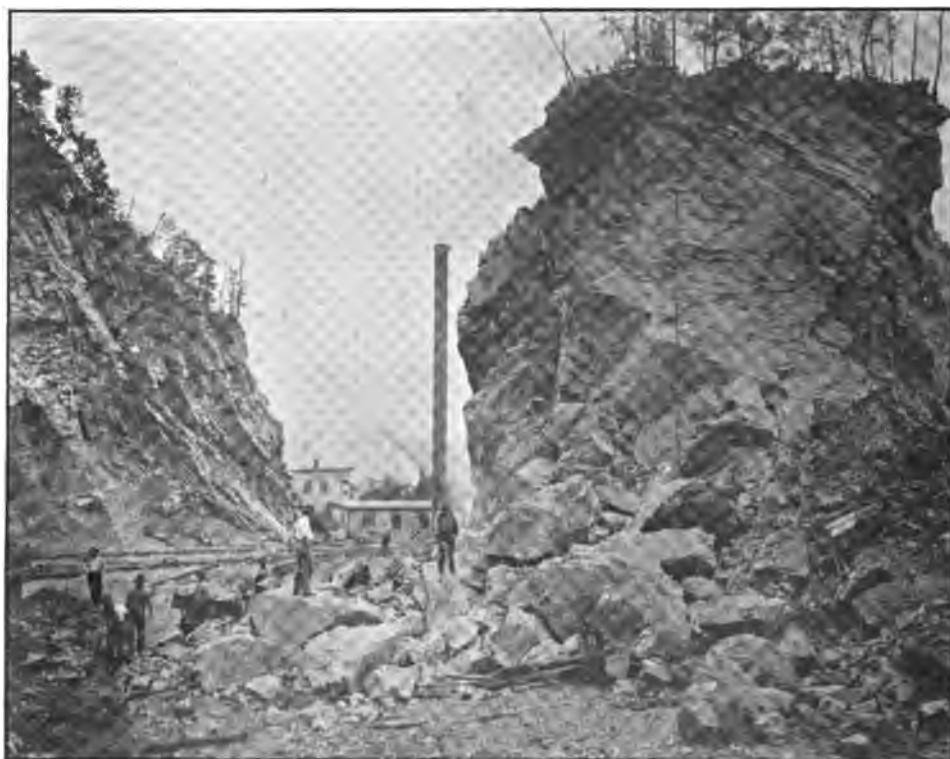
B. First quarry opened. Blue limestone. 20 feet above railway track.—G. C. Buquo Lime Company, Hot Springs, N. C.
